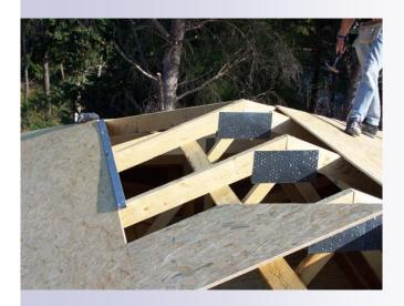
The roof truss is completely covered with so called OSB plates to guarantee an optimal protection against storms.
