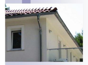
Another remarkable advantage is the roof overhang, which does not need any maintenance works (hard silicon plaster). Regular painting is not necessary, as the roof overhang has the same weather protection like the whole façade.
