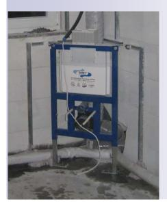
All the toilets have been made with a front-wall installation. The complete pipes for a convector heating system are already laid concealed. The bathrooms have electrical under-floor heating.
