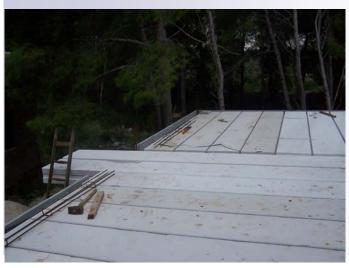
The ceiling to the upper floor is a prefabricated unit made in Germany.
