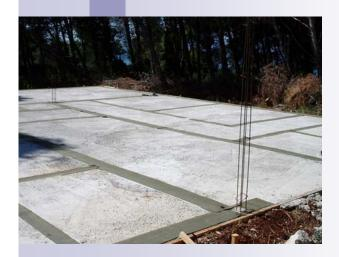
The house is founded with ca. 130 m<sup>3</sup> of concrete and two layers of steel on Brac's marble ground.
