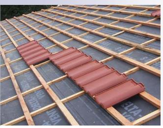
The big roofing tiles are held together by staples and are therefore very well protected against storm. Also, a waterproof but permeable sarking membrane has been installed to guarantee best protection against moisture.
