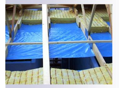
A vapour barrier on the upper floor provides for perfect dryness in all the insulated rooms. Therefore, the persistency of the roof construction is guaranteed.
