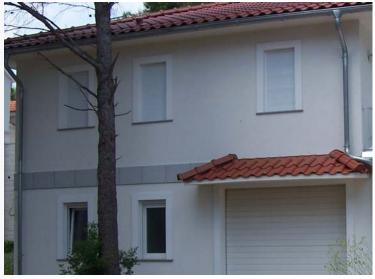
All the window sills as well as the stairs and the foundation of the façade are made of very durable, easy-to-clean granite.
